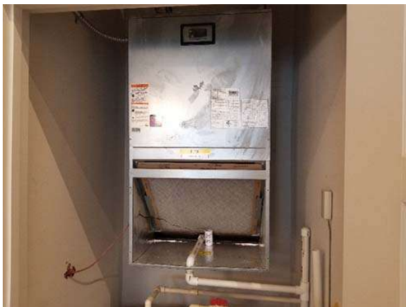
Typical residential type AHUs may not be suitable for high efficiency MERV-13 or above filters. Verify the AHU performance including ductwork layout to determine if such filters are suitable for its intended application.
