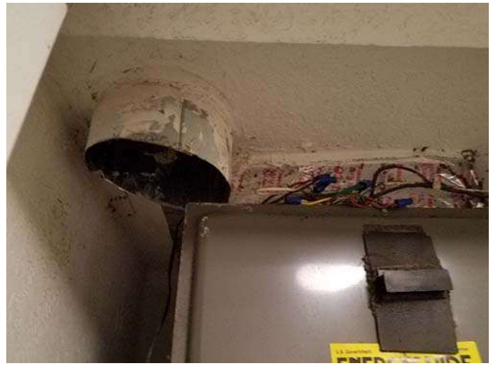
Photo of outdoor air duct stubbed into apartment AHU plenum closet. Not ideal but would be better to duct down to return air opening of AHU and provide volume damper for control.
