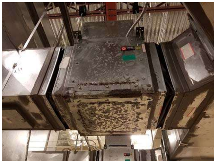
Example of excessive non-conditioned outdoor air effects into an outdoor air fan/duct system causing deterioration and corrosion of surrounding equipment and materials
